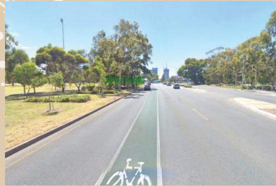
Vehicle approach view from approximately 100m to the proposed Kurna Welcome Installation site (shown in green)
