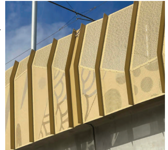
AUD- Tram Grade Separation Project
